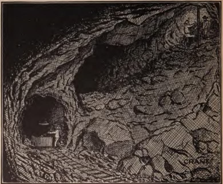
FIG. 5.—Overhand Stopping, 'Breaking-Through.'
